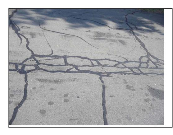
**Description:** Recently sealed cracks in asphalt paving
